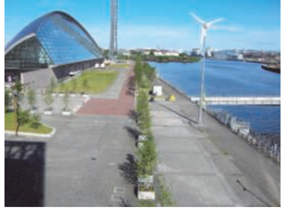
The Glasgow Science Centre—landscaping contract by Landscapes & Contracts Ltd
